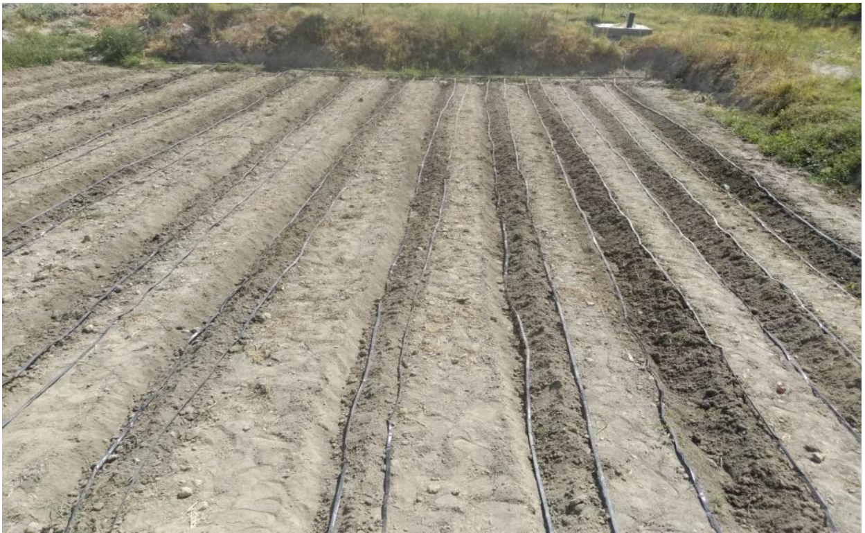
Figure 2. Installation of irrigation systems in the pilot field (2022)
