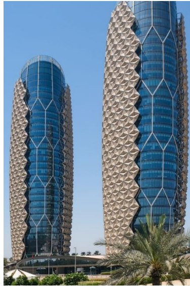
Fig. 2. Kinetic responsive facade of the Al Bahr Towers.
