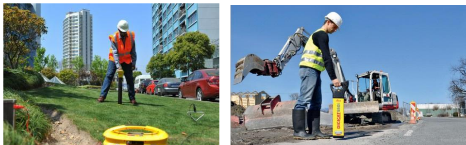
Figure 6. Practical use of pipe finders in the search of pipe networks
