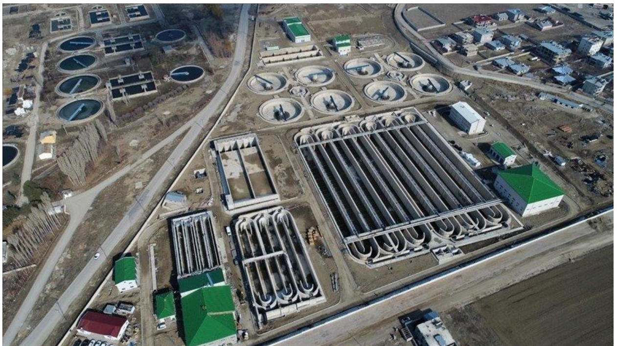
Figure 2. Turkey water treatment plant
