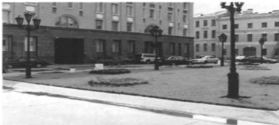
Figure 5. A used roof over an underground garage in St. Petersburg
